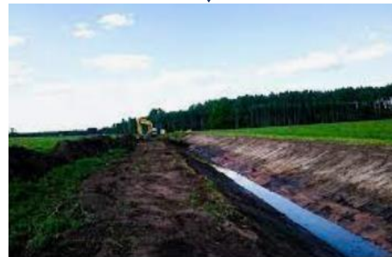
Excavation of ditches and ponds
