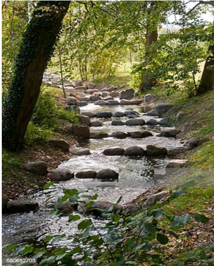
Figure 3.2.1. Bypass channel in Estonia
