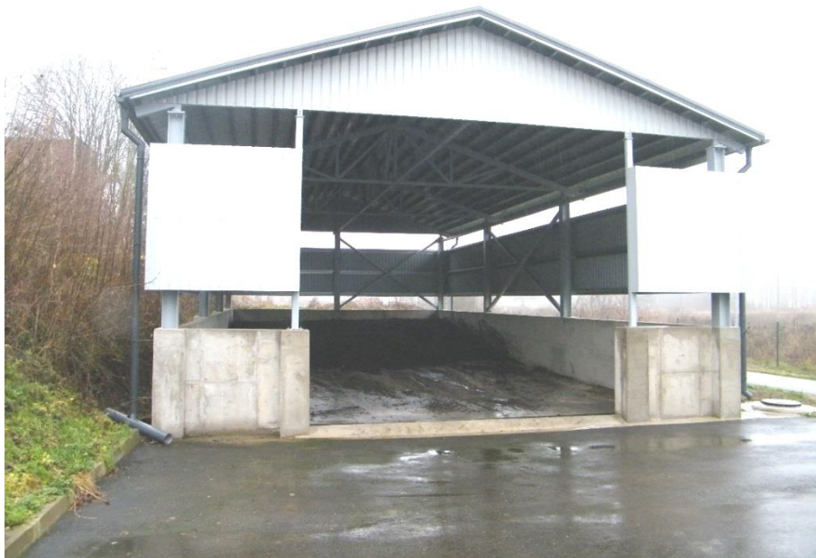
Figure 7.11 Dewatered sewage sludge storage shed. Considered to be no source of CH 4 emissions
