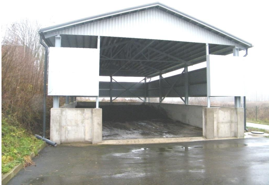
Figure 7.11 Dewatered sewage sludge storage shed. Considered to be no source of CH 4 emissions
